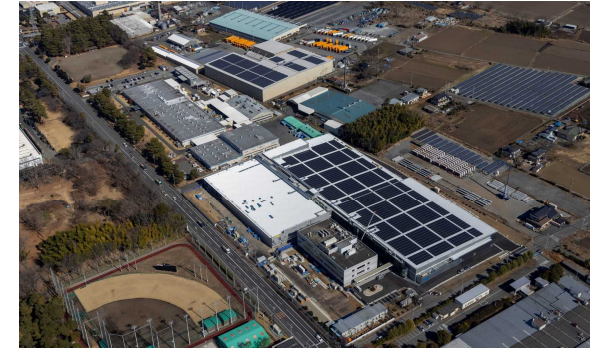
Solar panels on new Moka Plant
