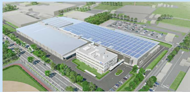
Solar panels on new Moka Plant
