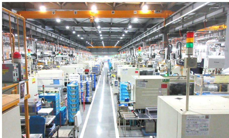
Interior of the new plant
