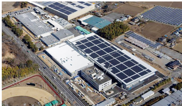
Solar panels at the new Moka Plant
